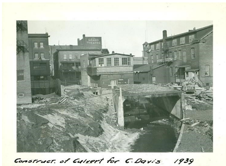
Figure 5 – The construction of box culverts in Downtown Sudbury, 1939. Photo from Conservation Sudbury.
